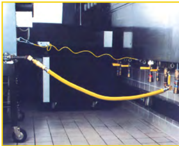
Usable length of hose with SwiveLink
